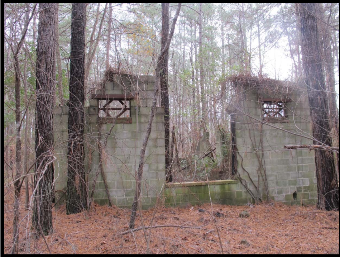
ED1651 – View of Commercial Building, 12601 NC 97 West, Looking Southeast.
