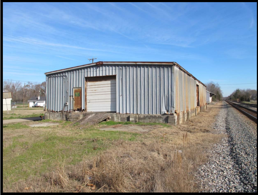
NS1551 – View of Depot/Warehouse, Railroad Street, Looking Northwest.
