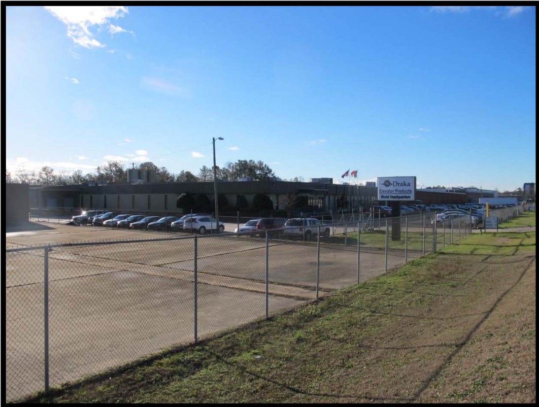
NS1546 – View of Commercial Building, 2151 Church Street, Looking Southeast.
