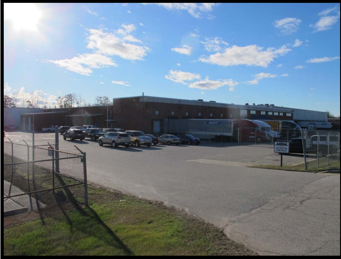
NS1547 – View of Commercial Building, 1951 Church Street, Looking Southeast.
