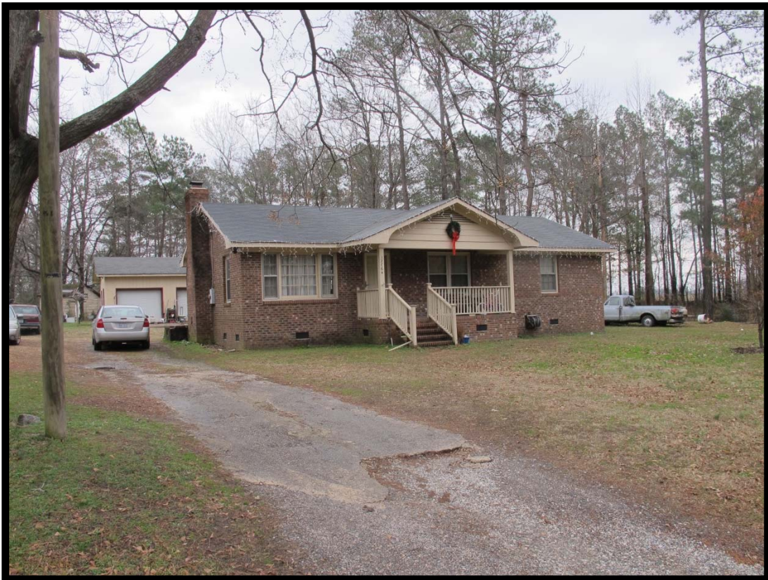
NS1540 – View of House, 12664 Center Street, Looking Northeast.
