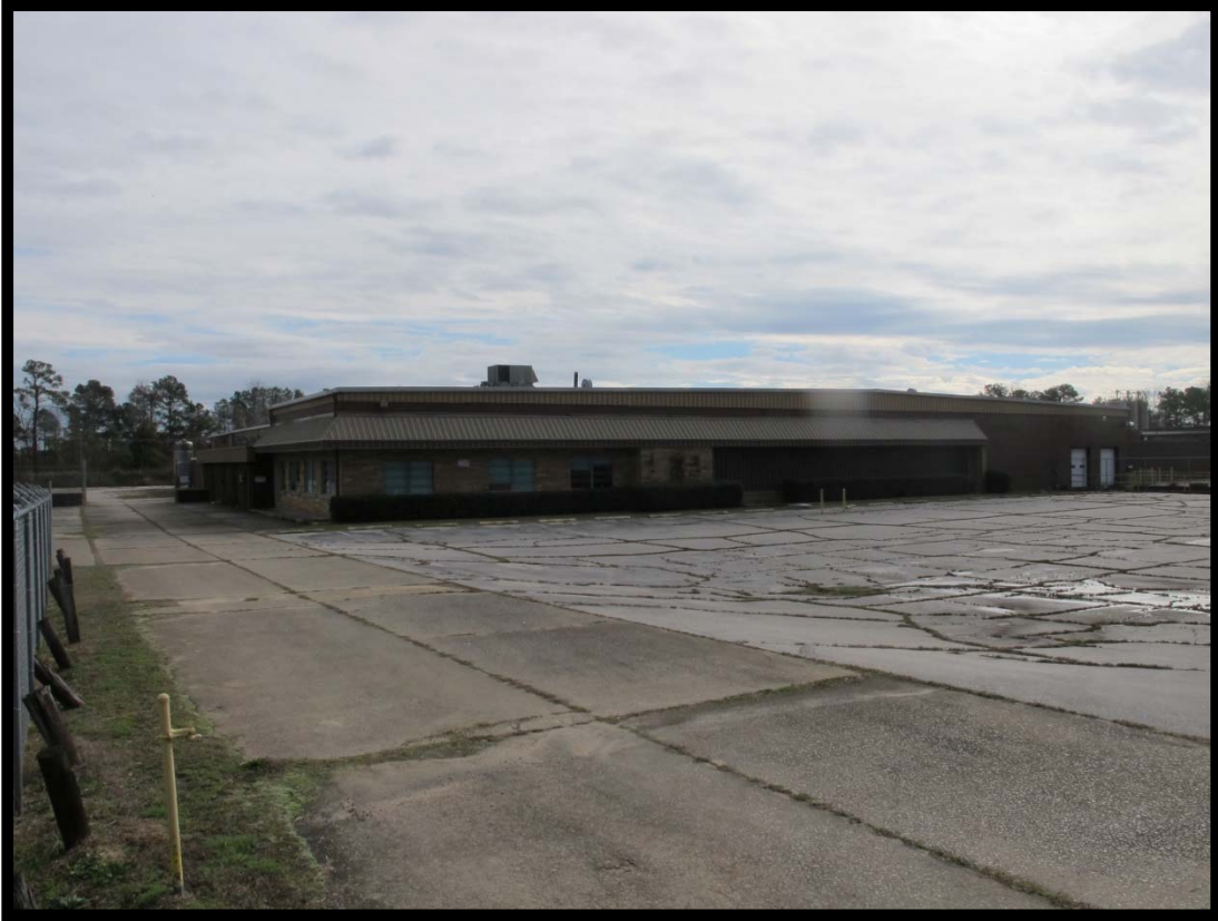
NS1545 – View of Commercial Building, 2245 Church Street, Looking Southeast.
