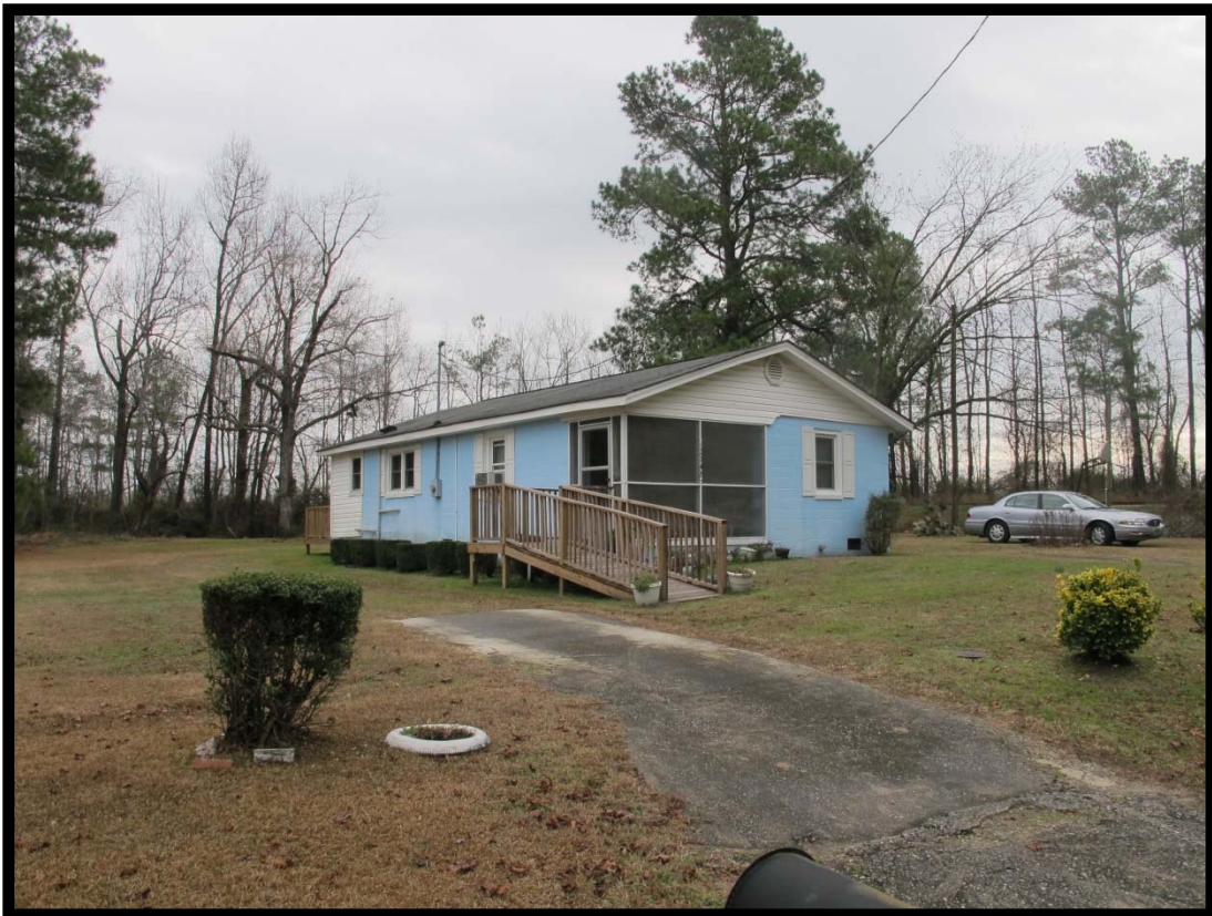
NS1542 – View of House, 12748 South Street, Looking Northeast.
