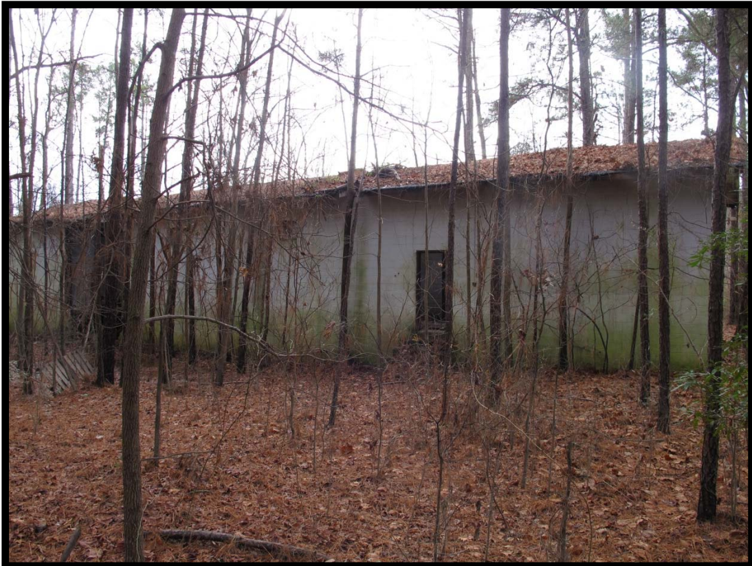
ED1651 – View of Commercial Building, 12601 NC 97 West, Looking Southwest.
