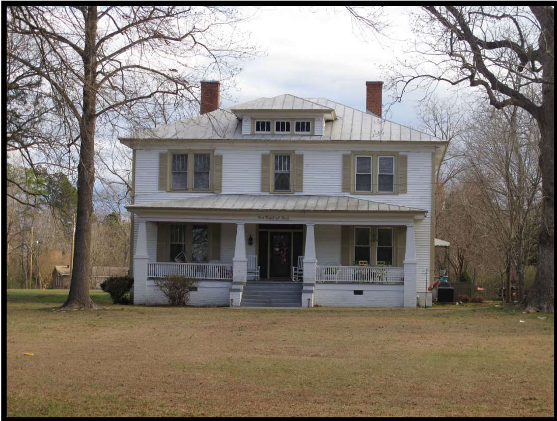
ED1654 – View of House, 104 E. Battleboro Avenue, Looking North.
