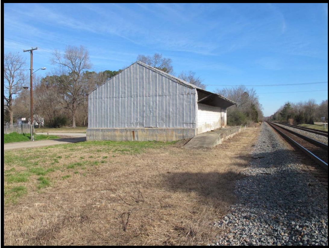
NS1550 – View of Depot/Warehouse, Railroad Street, Looking Northwest.
