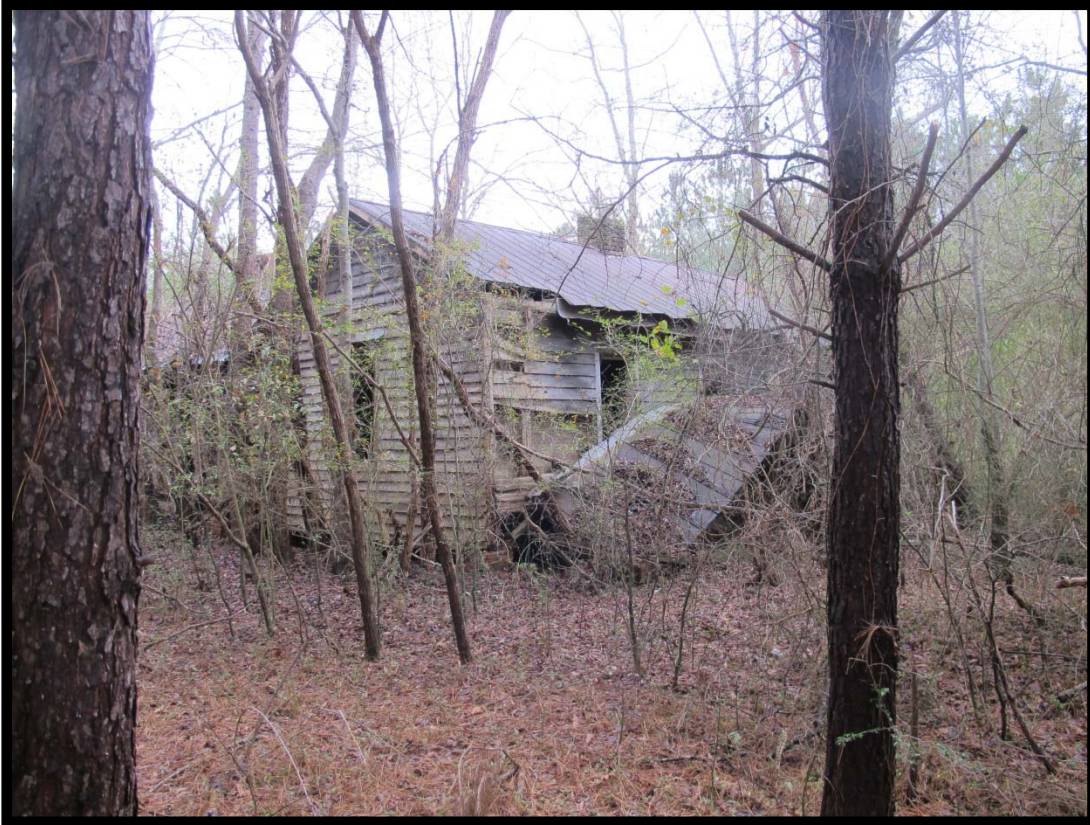
ED1648 – View of House, Berrywood Lane, Looking South.
