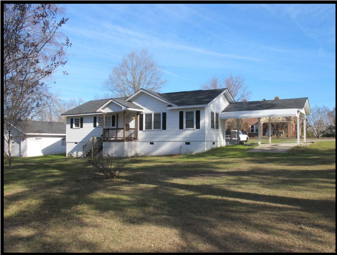
NS1552 – View of House, 104 Etheridge Street, Looking North.
