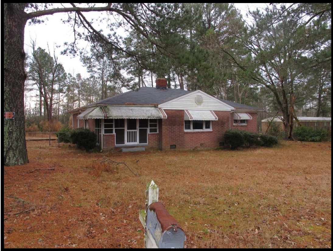
NS1541 – View of House, 10891 East Street, Looking Southeast.
